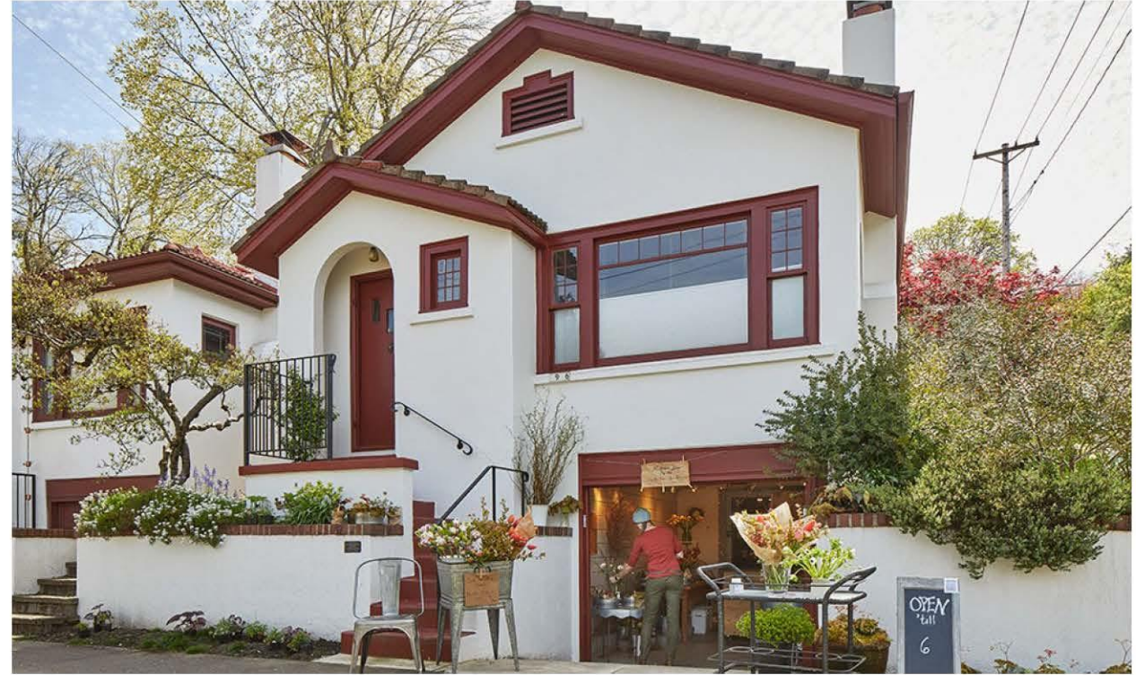
Bohnsen Cottage, a Historic Landmark with garage converted to a flower shop
