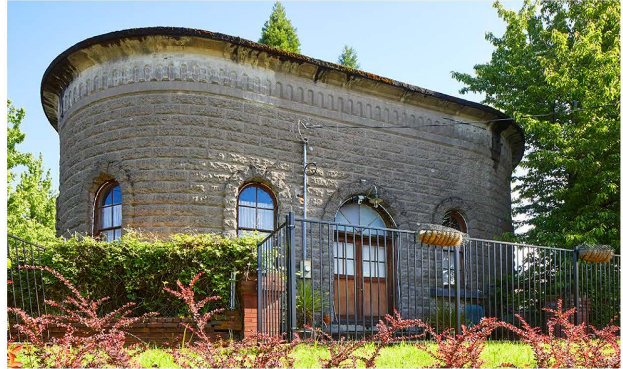
Portland Reservoir #2 Gatehouse, a Historic Landmark converted to a single-family house
