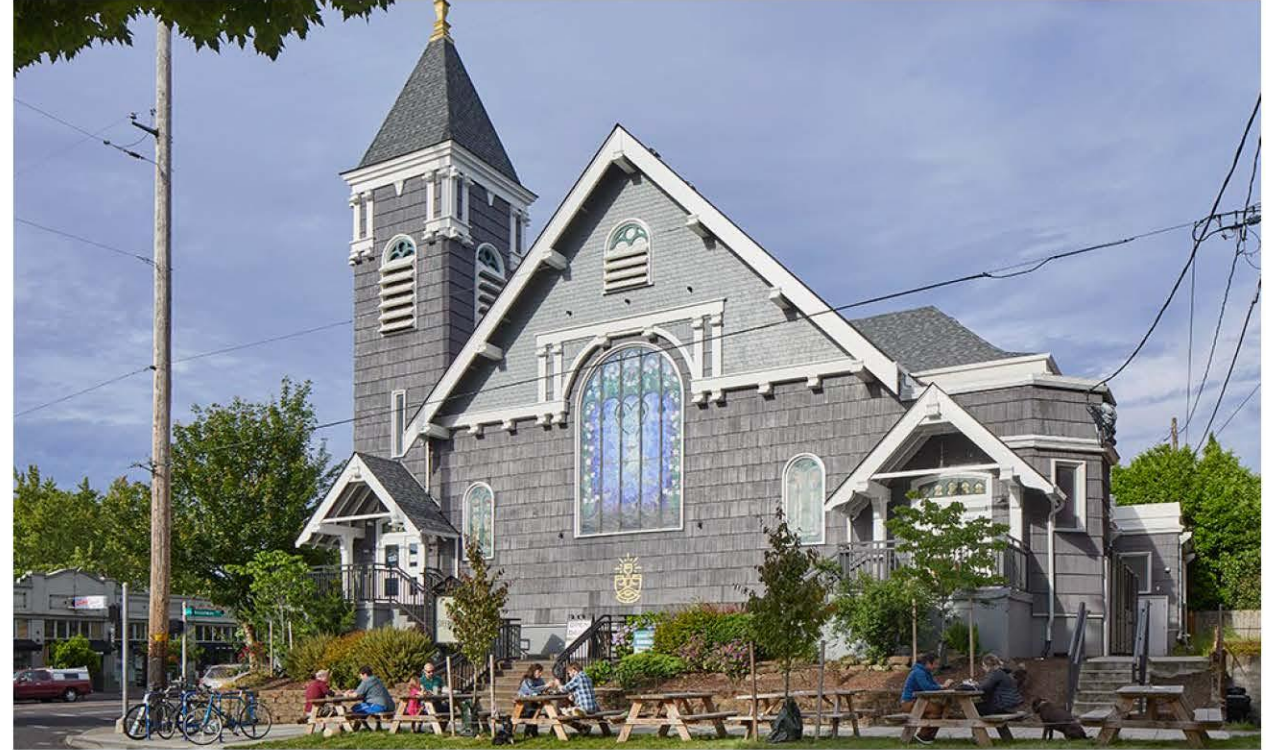
Metropolitan Community Church, a Significant Resource now used as a brewery and event space
