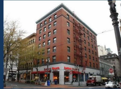
Whitmarsh Bldg, Downtown Portland
