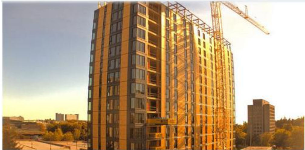
Uncommon ground: At 18 floors, Vancouver's Brock Commons will be the world's tallest wood-framed structure in 2017.
